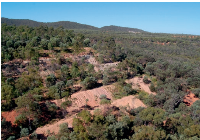
Fig. 3. Aerial photo of a rehabilitated waste rock dump (Au mine, Australia), showing an exposed, barren sulphide-rich layer on an outer dump batter. A flawed repository design, inadequate waste characterisation and poorly supervised waste management practices led to today's physical instability of waste rock batters, ineffective encapsulation of potentially acid-forming (PAF) materials, exposure of PAF materials, and resultant erosion, vegetation dieback and impacts on ground and surface waters.
